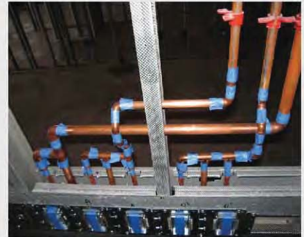
Conventional gas piping requires multiple connections as seen by blue tape leading to increased costs.
