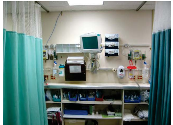
After Nexspan Equipment Rails Installed
